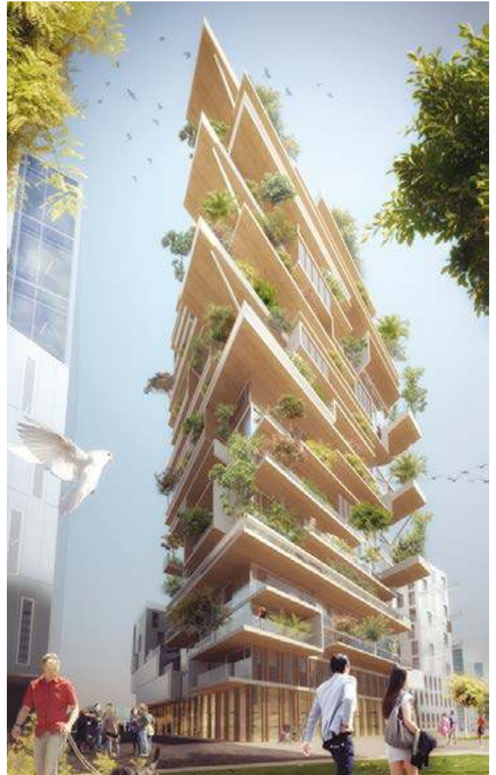
An 18 storey CLT apartment complex in Bordeaux France.
